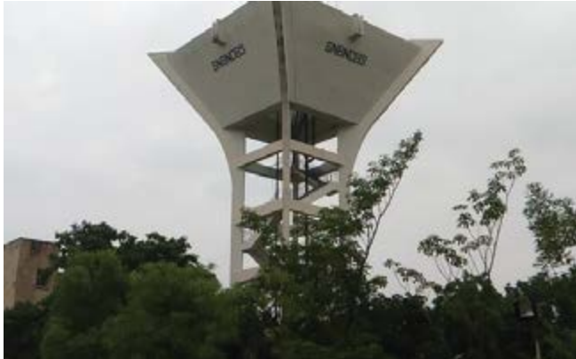
RCC Overhead Water Tank
