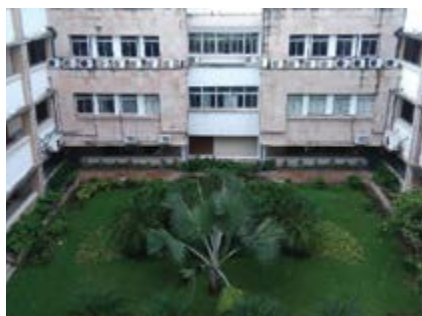
Main Building internal Courtyard
