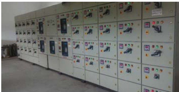
Electrical Panels in New Sub Station
