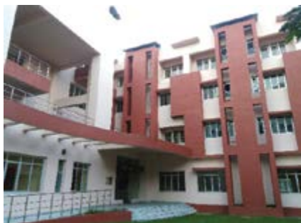
IHB&TQC Building Front View
