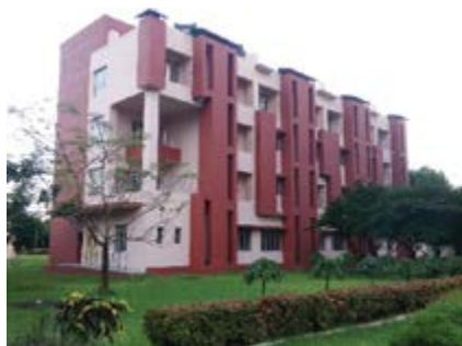
IHB&TQC Building Side view
