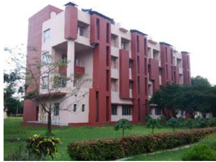
IHB&TQC Building Side view
