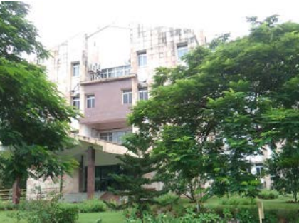
Main Building (Front)
