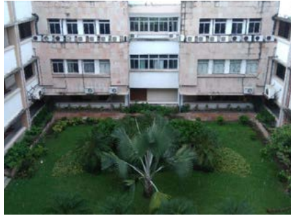
Main Building internal Courtyard
