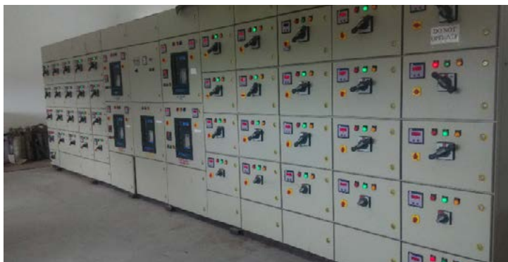
Electrical Panels in New Sub Station
