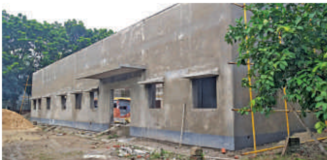
Lab Building under Construction
