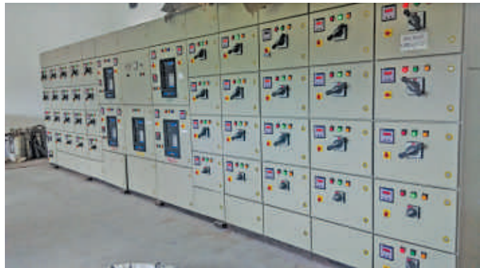
Electrical Panels in New Sub Station
