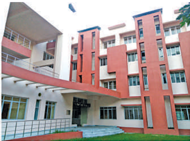
IHB&TQC Building (Basundhara) Front View
