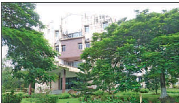
Main Building (Front)
