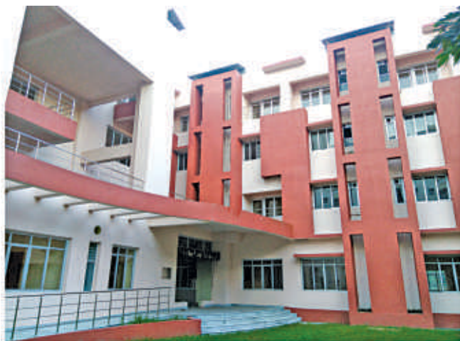
IHB&TQC Building (Basundhara) Front View
