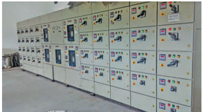
Electrical Panels in New Sub Station
