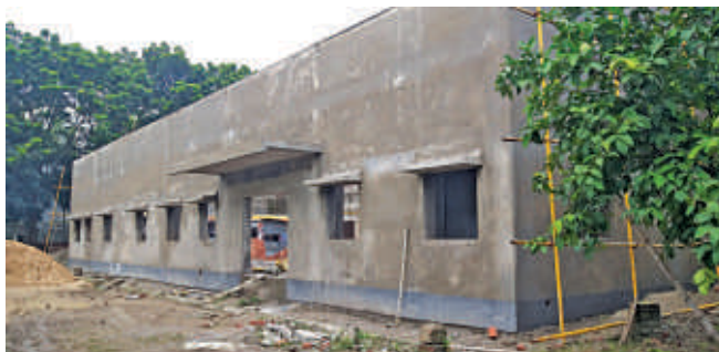
Lab Building under Construction
