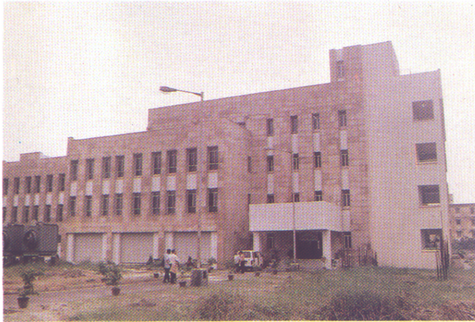
Main Building where the Library, Laboratory, Computer Room are currently housed
